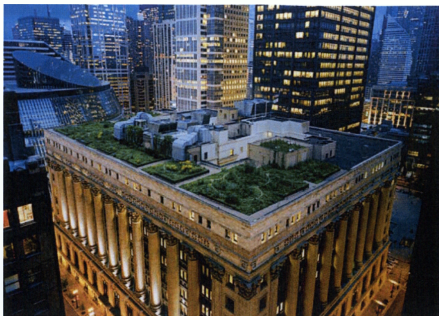
Εικ.27 Chicago City Hall green roof
